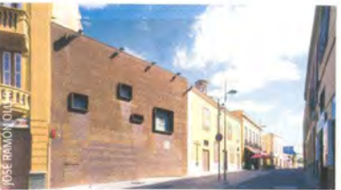
3 CAR PARK FOR BINGO PREMISES Architects: José Manuel Rodríguez Peña Completed: 2004 Address: Calle Candelaria, Plaza de la Iglesia, Santa Cruz de Tenerife
