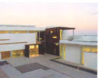
15 CONTINUOUS SERVICE CENTRE Architects: e4 quevedo & fdez-palacios, Ana Fdez-Palacios Martínez, Alberto Quevedo Domínguez, Víctor Quevedo Domínguez, José J. Quevedo Domínguez Completed: 2005 Address: Calle Mijail Gorvahov, Carrizal, Ingenio
