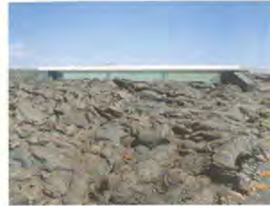
25 RESIDENCE-WORKSHOP CÉSAR MANRIQUE FOUNDATION Architects: Juan Manuel Palerm Salazar, Leopoldo Tabares de Nava y Marín Completed: 2004 Address: Taro de Tahiche, Lanzarote
