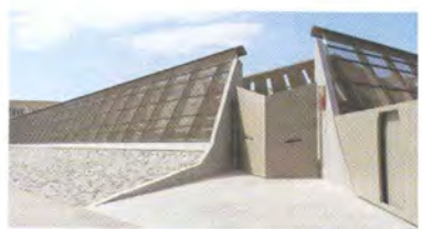
17 INFANT WING OF NESTOR ALAMO STATE SCHOOL Architects: Manuel J. Feo Ojeda, Juan J. Espino Duran Completed: 2003 Address: Rambla de Jinamar, Las Palmas de Gran Canaria
