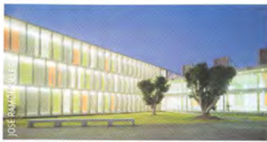
6 MARINA CEBRIÁN SECONDARY SCHOOL Architects: GPY arquitectos, Juan Antonio González Pérez, Urbano Yanes Tuña Completed: 2004 Address: Calle Candelaria s/n, Taco, La Laguna
