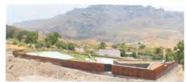
16 SANTA LUCÍA COUNCIL SWIMMING POOL Architects: e4 quevedo & fdez-palacios, Ana Fdez-Palacios Martínez, Alberto Quevedo Domínguez, Víctor Quevedo Domínguez, José J. Quevedo Domínguez Completed: 2005 Address: Santa Lucía casco, Santa Lucía
